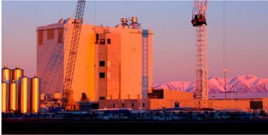
Darfield site during construction Courtesy - Fonterra Co-Operative Group
